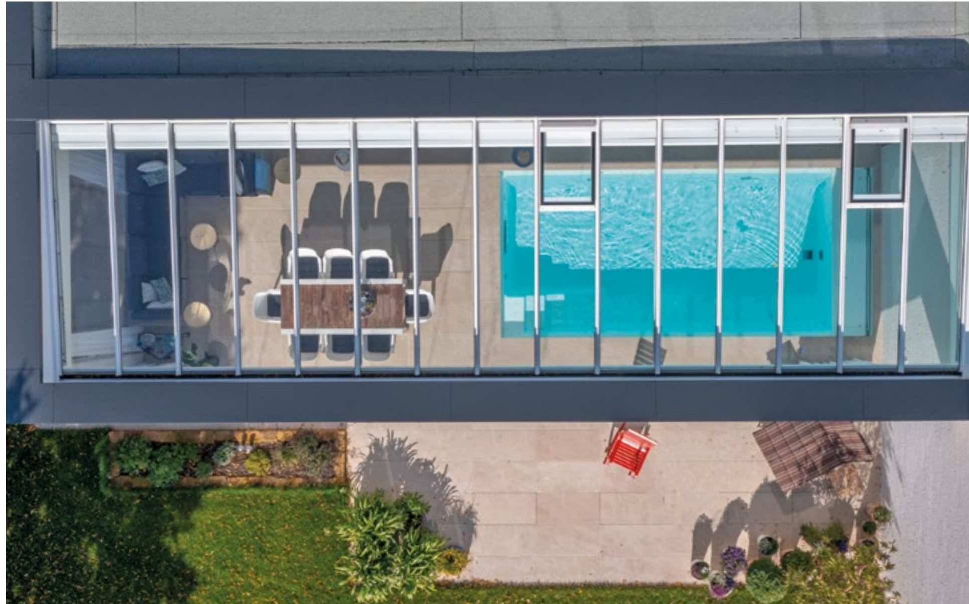
AirSlide- Riviera Pool, Wintergartenzentrum Münsterland
